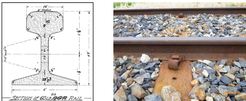
**Figure 14** Visually comparing new and existing rail head depths for wear
