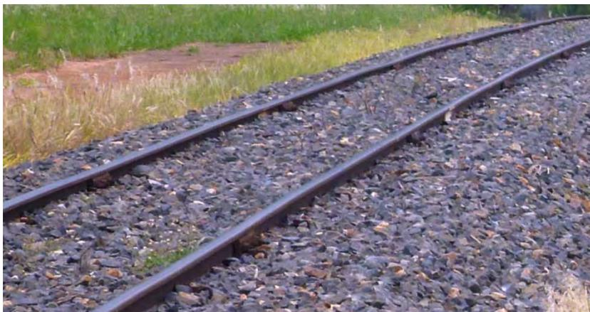
**Figure 13** Poor longitudinal surface smoothness because of frequent rail joints
