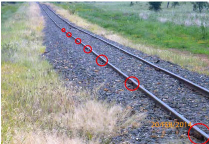
**Figure 12** Very short rail lengths between fish-plated joints. 24ft (7.3m)
