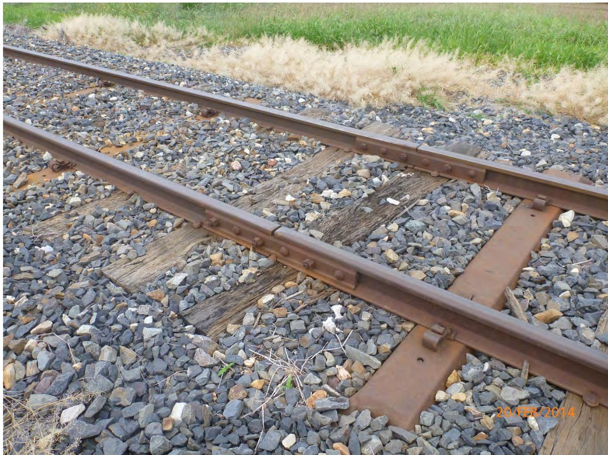
Figure 2 Timber sleepers interspersed with steel sleepers (1 in 4) - Central West System
