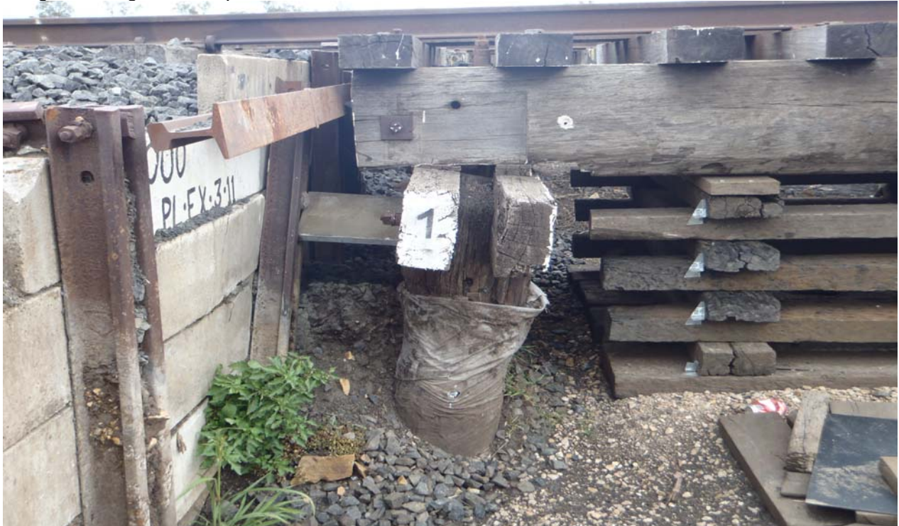
Image 3: Bridge to be replaced at the 84km mark
