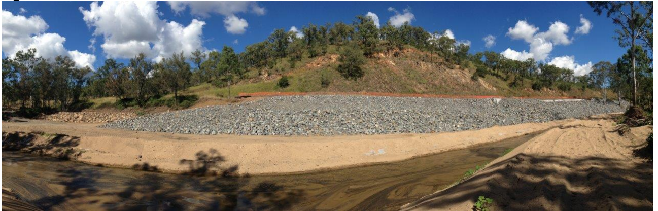
Figure 13 Reconstructed embankment with rock fill and reinstated Bells Creek
