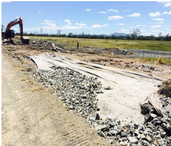
Figure 8 Track panel removed at Clarke (61.22km)
