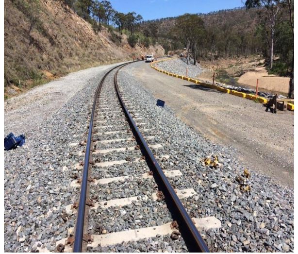
Figure 3 Re-slewed track to permanent location
