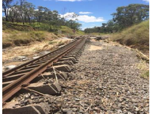
Figure 9 Earlsfield–Dakenba (15.07 Km) washout
