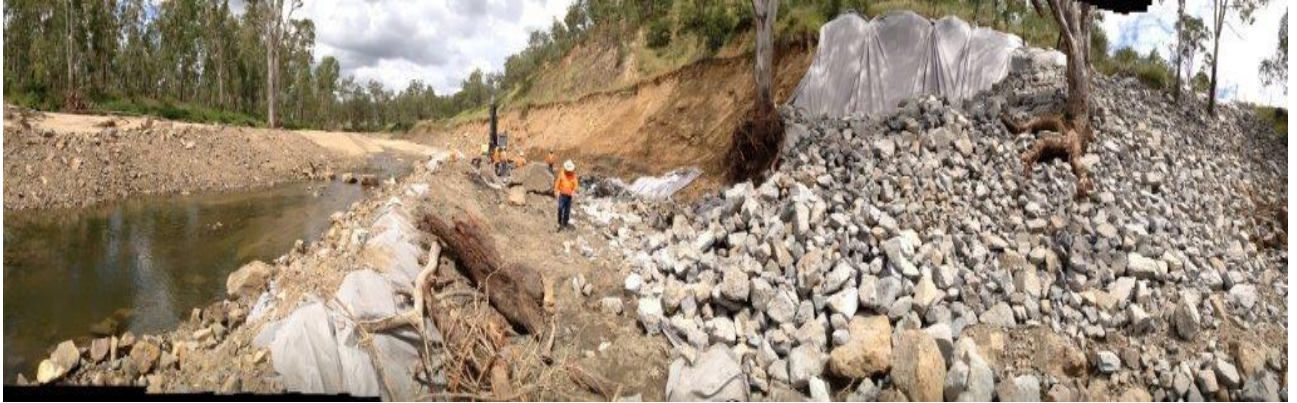
Figure 12 Reinstatement of embankment at Bells Creek
