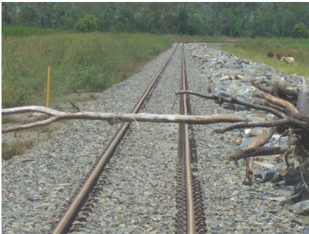
Figure 4 Track protected by flood rock
