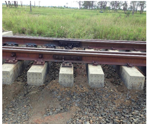
Figure 9 Earlsfield–Dakenba (15.07 Km) washout
