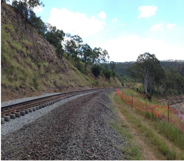
Figure 2 Slewed track to temporary location
