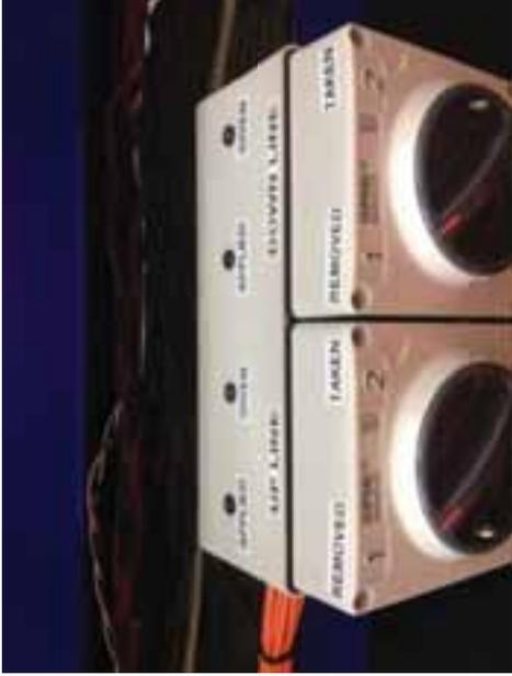
Activated via control switch on-site by track protection officer.
