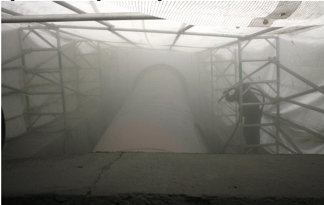
Figure 10.8: Pipeline after Re-Coating Works
