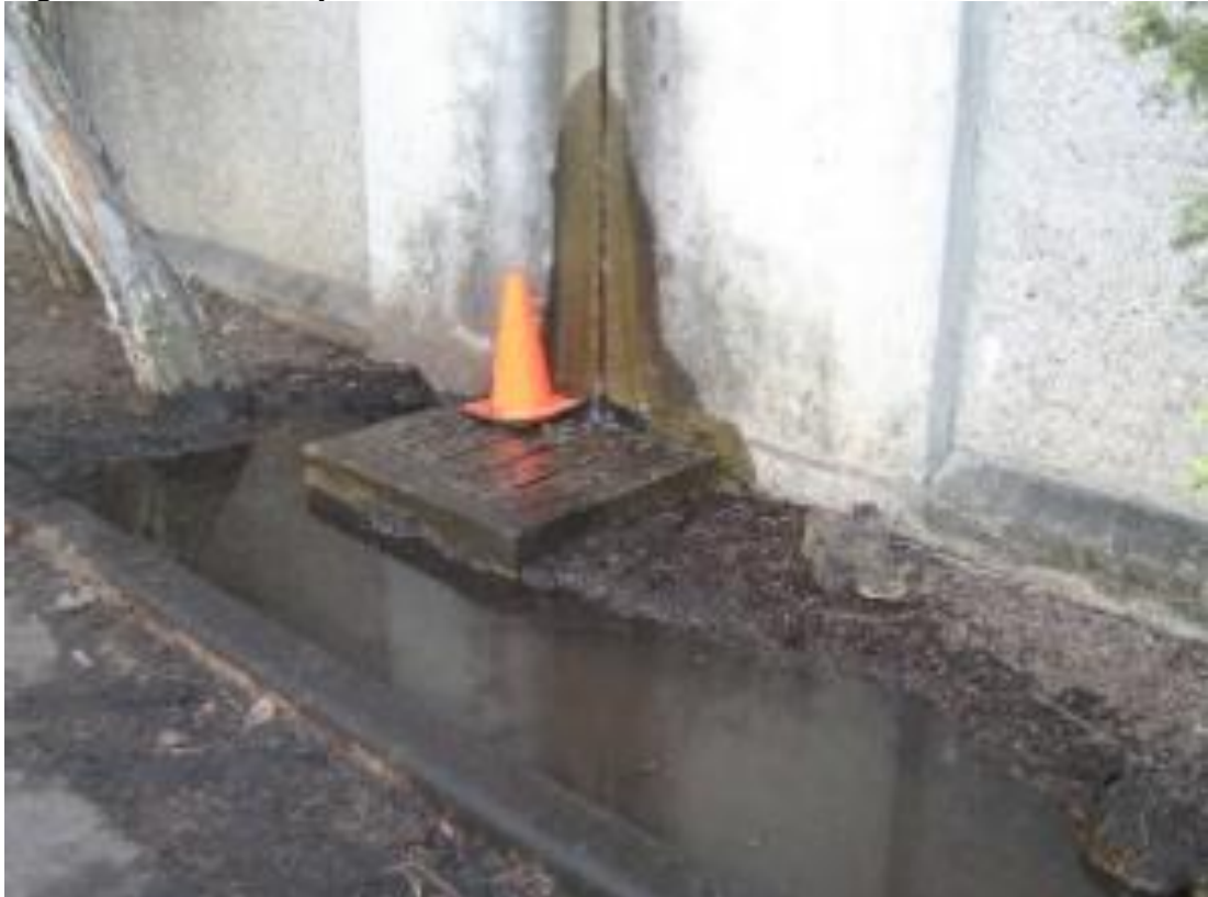
Figure 10.4: Wall Expansion Joint Leaks
