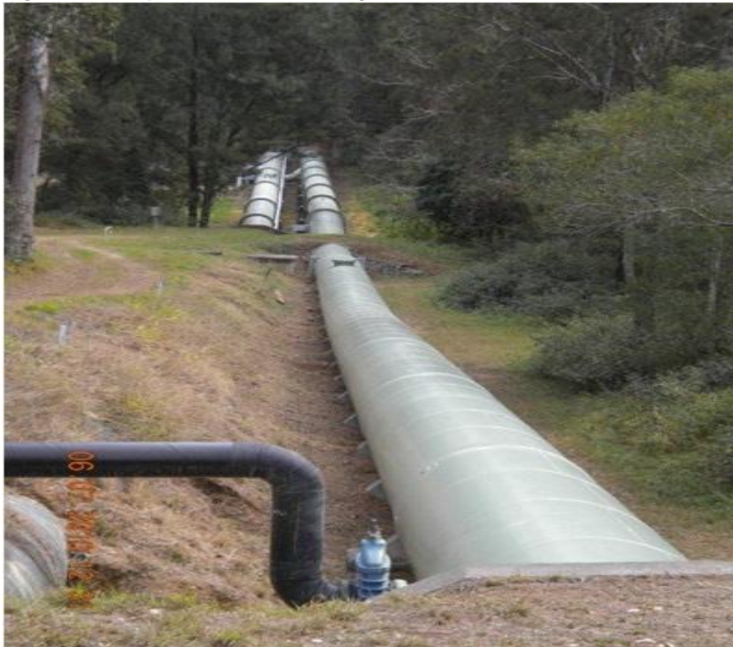
Figure 10.8: Pipeline after Re-Coating Works
