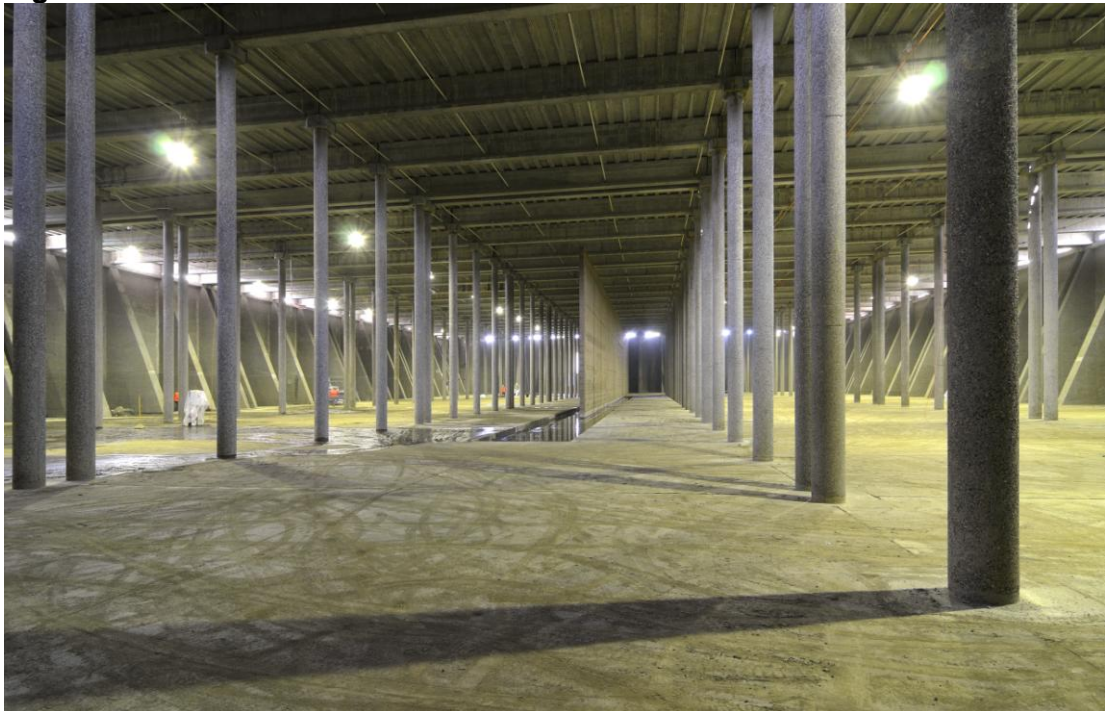
Figure 10.5: Reservoir Drained for Internal Refurbishment Works
