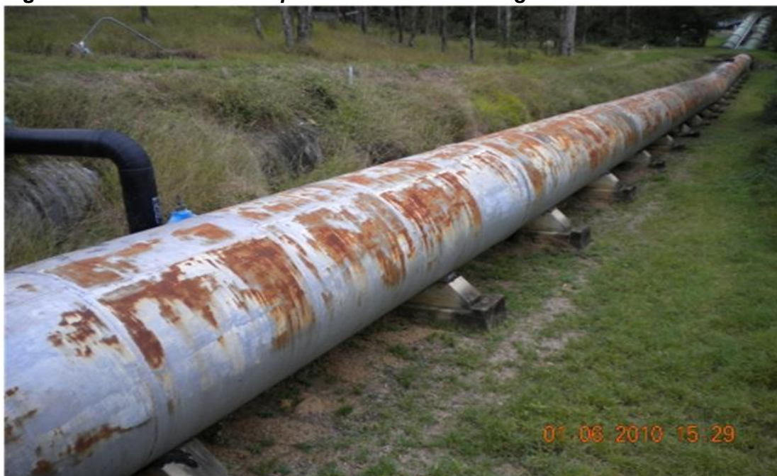
Figure 10.6: Condition of Pipeline before Re-Coating
