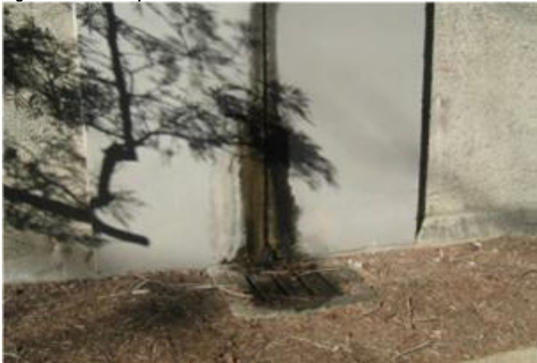
Figure 10.3: Wall Expansion Joint Leaks
